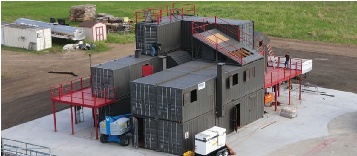
Conex Burn Prop Completed in 2020
